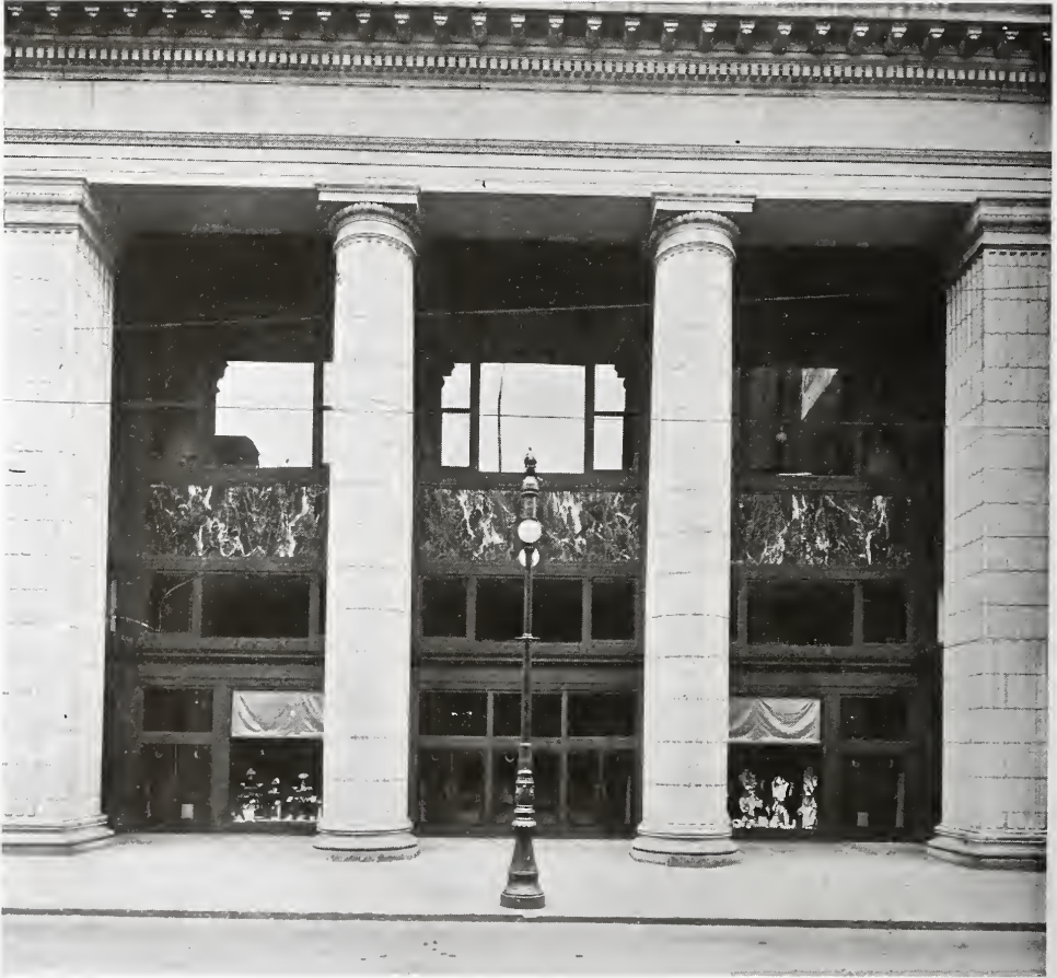
ENTRANCE DETAIL—THE WANAMAKER BUILDING.
